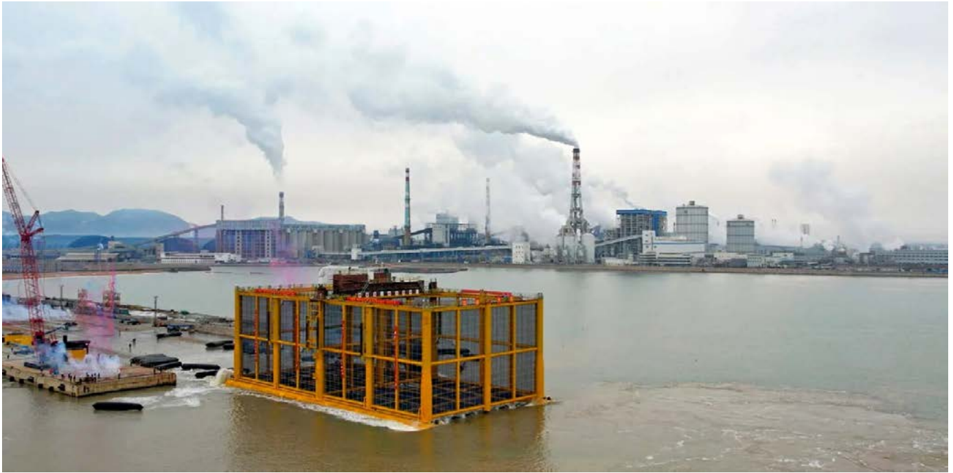
Sea Granary No. 1' in China. Has an annual output of 1,000 metric tons of Atlantic salmon. The cage is 35.9 meters high, 89 meters long. @Wanzefeng Group
