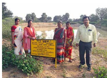
A step pond and embankment at Seja village, block- Kasipur, dist-Purulia. Photo: DRCS
