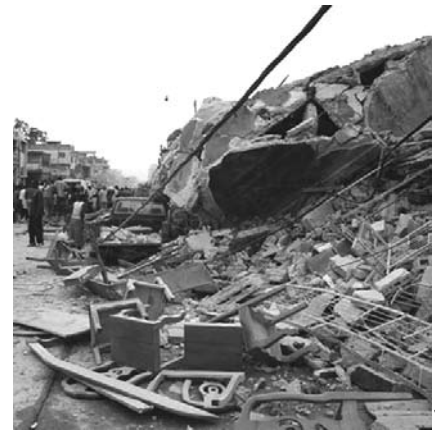
Earthquake damage, Port-au-Prince, Haiti, January 2010
