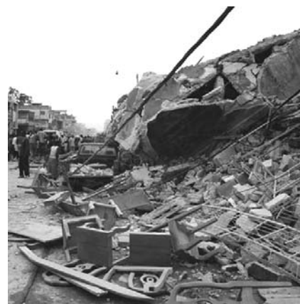
Earthquake damage, Port-au-Prince, Haiti, January 2010
